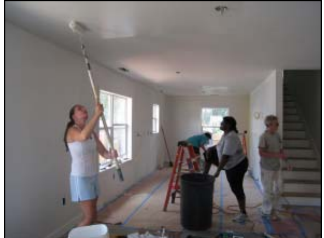
Melissa, Wanda and Gwen finishing up the kitchen.
