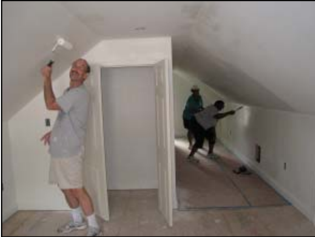
Bob, Wanda and Gwen working in the upstairs bedroom.
