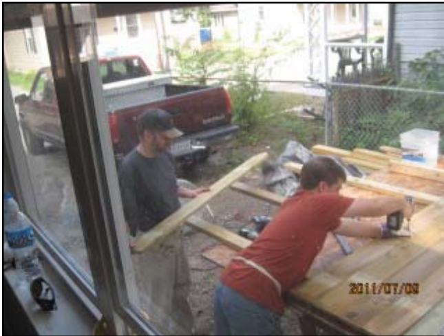
David and his son using power tools to build the fence.
